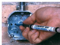
The picture shows the Condrive 1000 Installation Kit in action. The kit makes for fast and easy change over from drill bit to driver and controls the driving torque to prevent thread stripping and head snapping in hard base materials.
