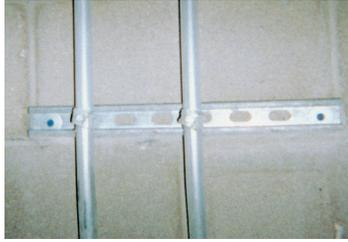
Many horizontal or "wall" applications are attached with Tapcon Anchor because it is removable and works well in block and brick.
