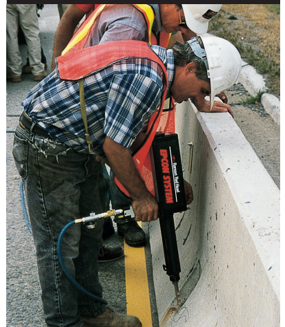
ANCHORING CONCRETE TRAFFIC BARRIER
